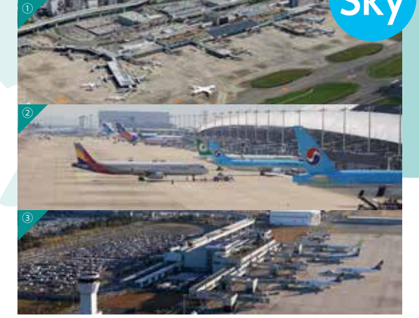
▲ ①Osaka International Airport ②Kansai International Airport ③Kobe Airport
